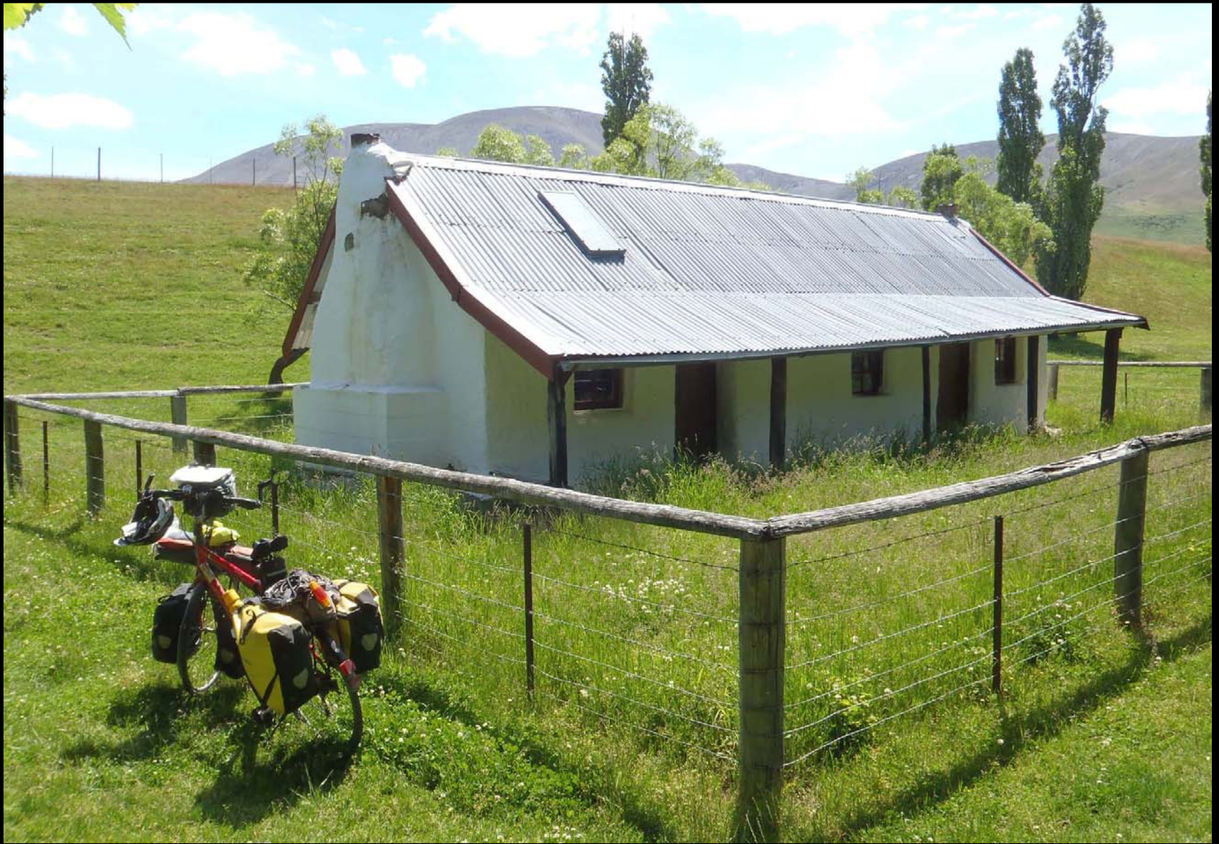
This is the Molesworth cob cottage, built in 1866 and used as accommodation for drovers who brought mobs of sheep across from Nelson to Canterbury 150 years ago. The walls of the cottage are a mixture of dried clay, dung and straw ("cob"). The roof was originally thatched with tussock, but that has now been covered with corrugated iron to reduce maintenance.
