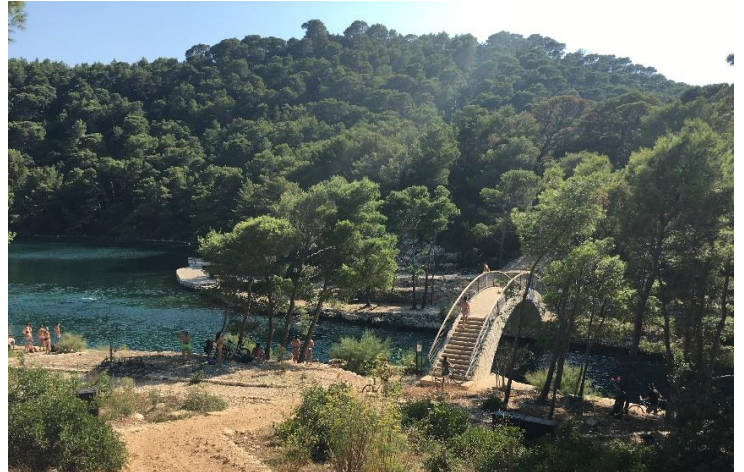
The arched bridge connecting both sides of the inlet
