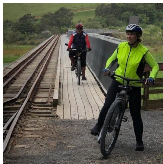
Taumarere Long Bridge
