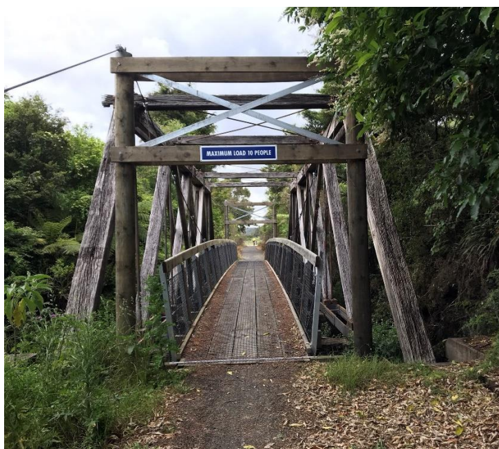
The interesting swing bridge constructed inside the old rail bridge
