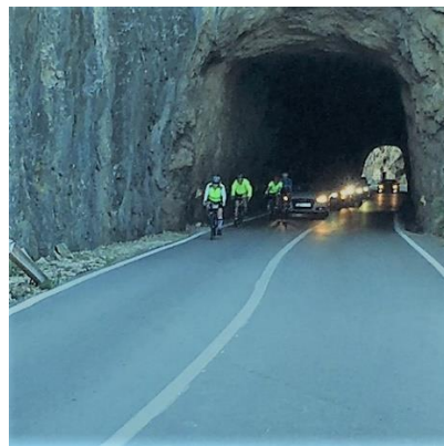
Riding up through tunnel
