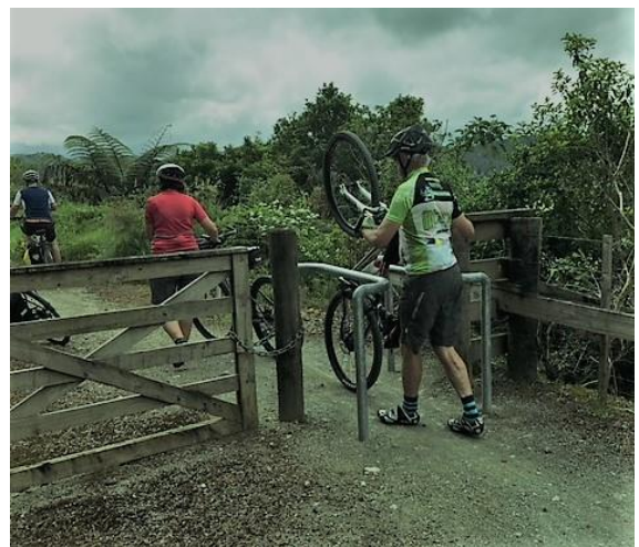
Having to “Stop and Start” going through cattle stops with bollards and cycle “squeeze bars” in order to prevent stock and motor bikes etc. entering the trail
