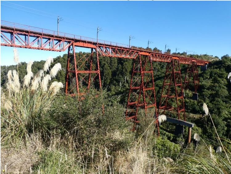
The Makatote Rail Viaduct
