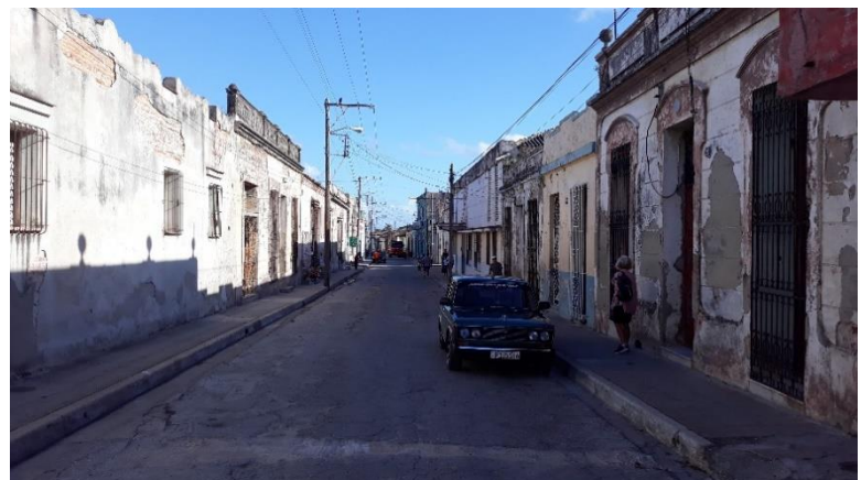
The state of buildings in a typical Cuban Town Street
