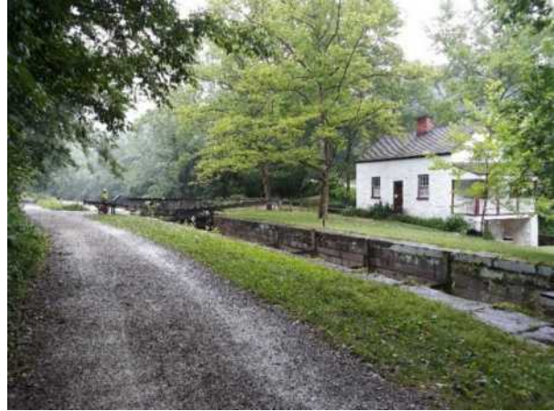
C and O Tow Path and canal control gate
