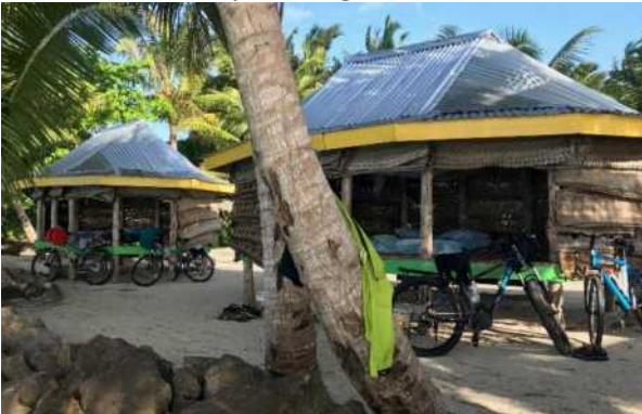
Fale Accommodation at Tanu Beach
