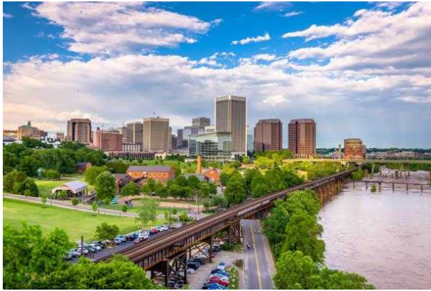
Left: Richmond and metal railway bridge
