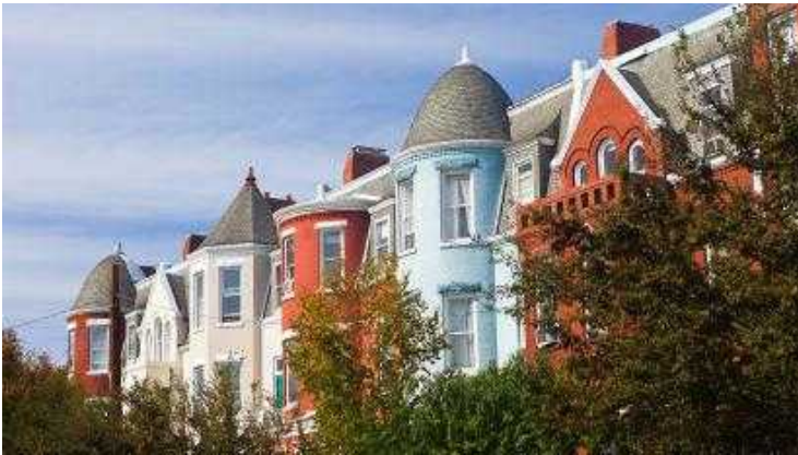
Left: Richmond Terraced Houses with Turrets
