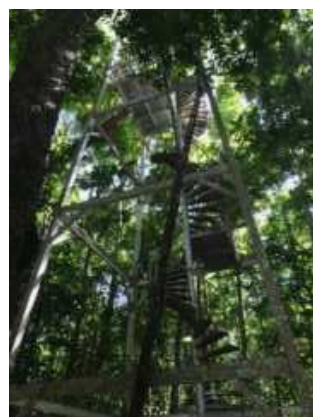
Stairs to the Canopy Walk
